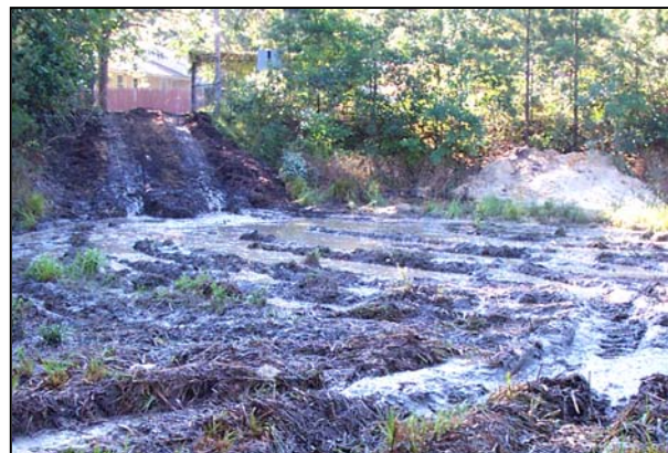
Stormwater basin at 11 th and Bismark Streets, Manchester Township, before restoration. Photo by Ocean County Soil Conservation District.
