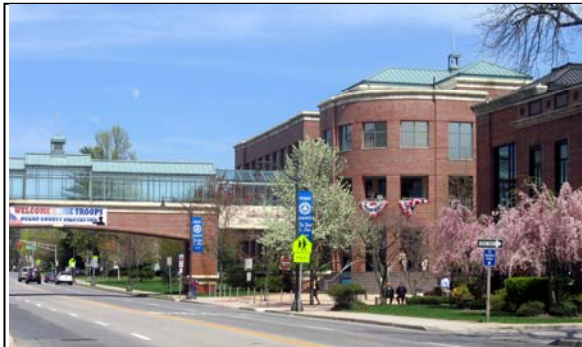
Planning, Engineering and Roads Annex at 129 Hooper Ave., Toms River, NJ. Photo by Ocean County Department of Planning.
