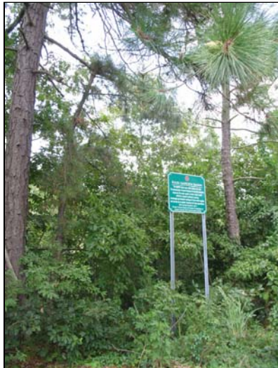
Restored stormwater basin in Manchester Township at 11th and Bismark Streets. The restoration eliminated flooding and mosquito problems. The basin has been completely revegetated. Photo credit: Ocean County Department of Planning.
